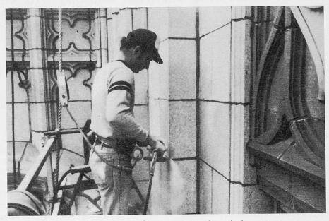
Fig. 7: Cutting of new expansion joints.
