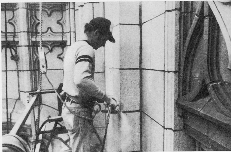
Fig. 7: Cutting of new expansion joints.
