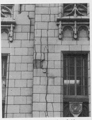
Fig. 2: Expansion failure
