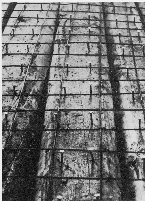
Fig. 4. The strengthening of a wooden ceiling under construction
