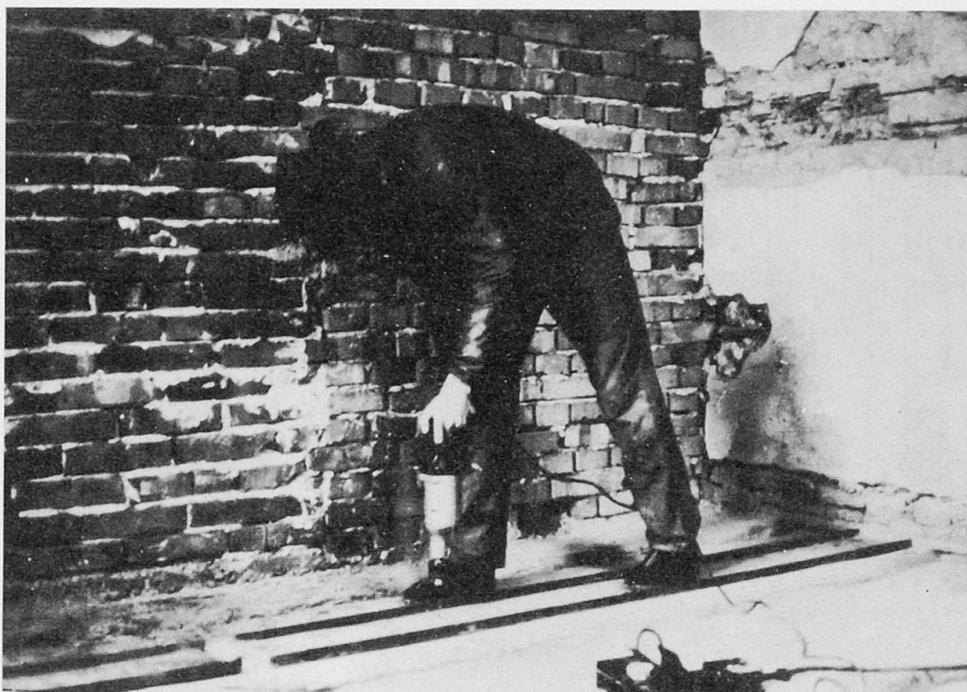
Fig. 6. Rough drilling with a drilling template
