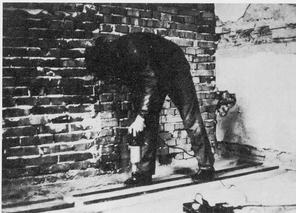
Fig. 6. Rough drilling with a drilling template
