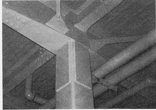
Fig.7 Coverplates welded
