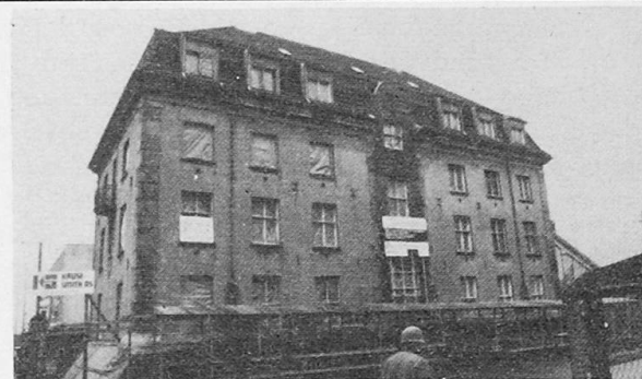
Fig.13. 2500 T being moved - Norway.
