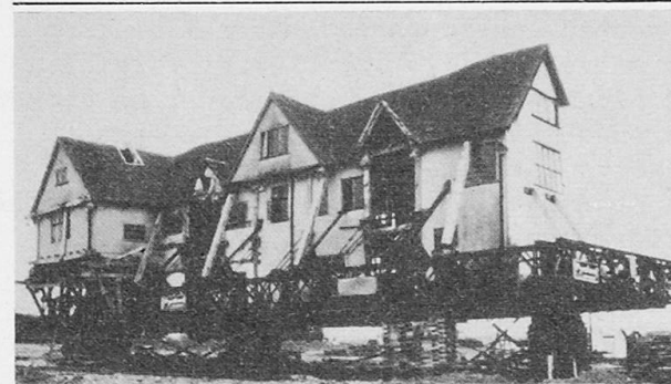
Fig.12. Steel frame under 17th Cent. mansion.
