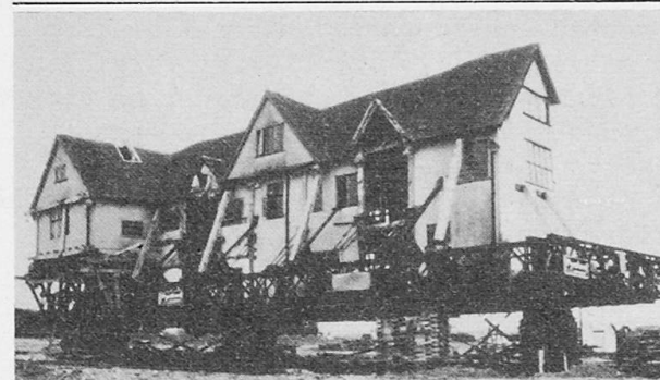
Fig.12. Steel frame under 17th Cent. mansion.
