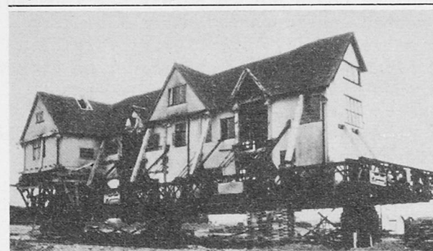
Fig.12. Steel frame under 17th Cent. mansion.
