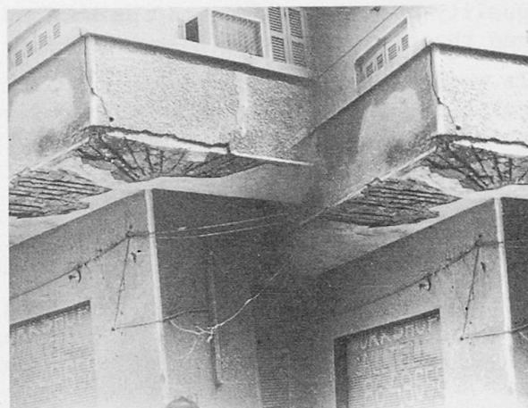
Fig. 6 Structure 2 showing concrete spalling due to rebar corrosion
