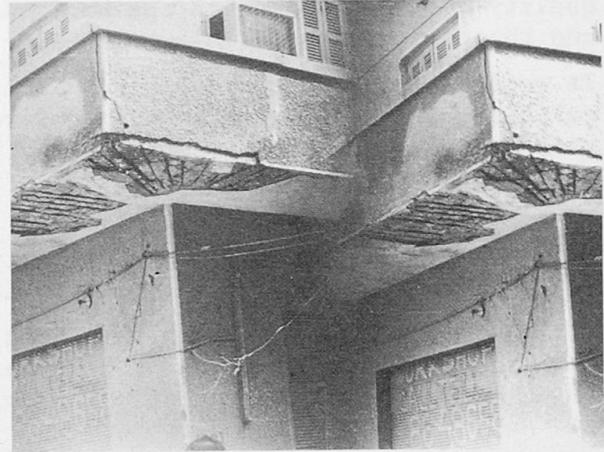
Fig. 6 Structure 2 showing concrete spalling due to rebar corrosion
