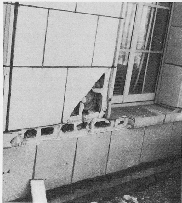
Fig. 4: Inspection opening
