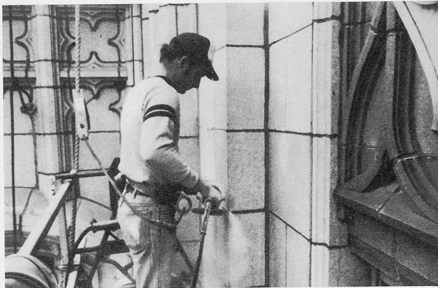
Fig. 7: Cutting of new expansion joints.
