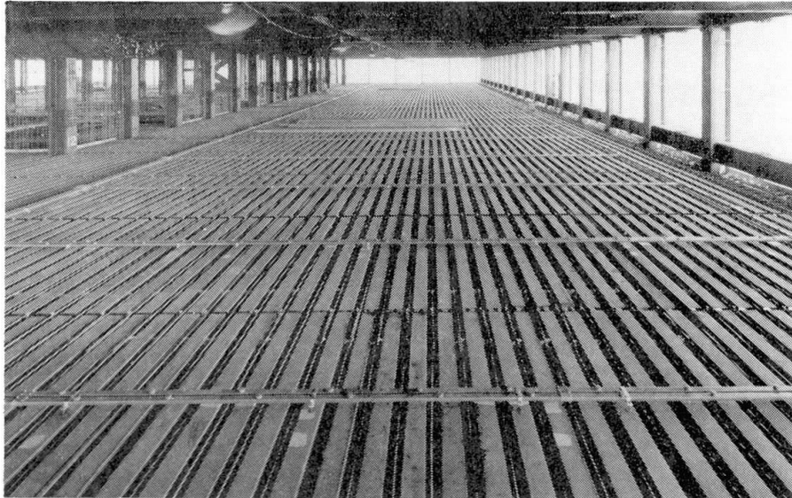
Fig. 6 One-way arrangement of bar and floor duct
