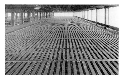
Fig. 6 One-way arrangement of bar and floor duct
