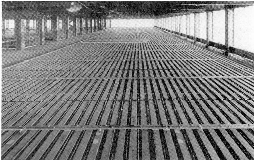
Fig. 6 One-way arrangement of bar and floor duct
