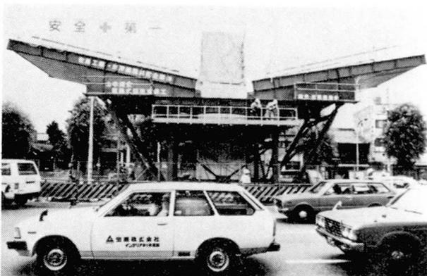
Picture 3. Construction beam for cross beam without any traffic disturbance
