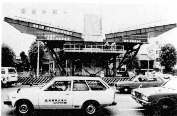
Picture 3. Construction beam for cross beam without any traffic disturbance
