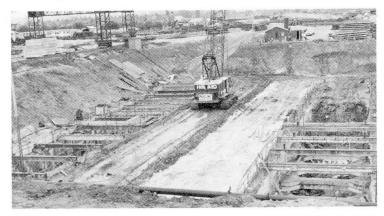
Excavation of the southern anchorage – strulting of longitudinal concrete walls.
