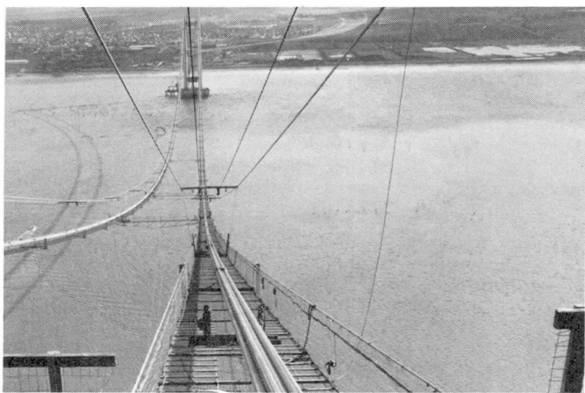
Mainspan cable part way through spinning process.
