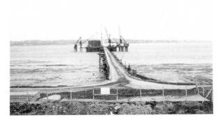
Construction of caissons at the end of the 500 m jetty.
