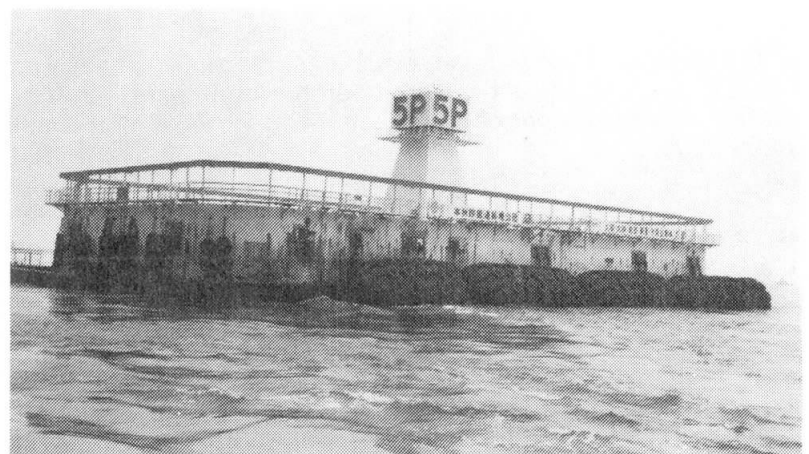
Fig.2 The Protection Installed on the No.5 Pier of the South Bisan-seto Bridge
