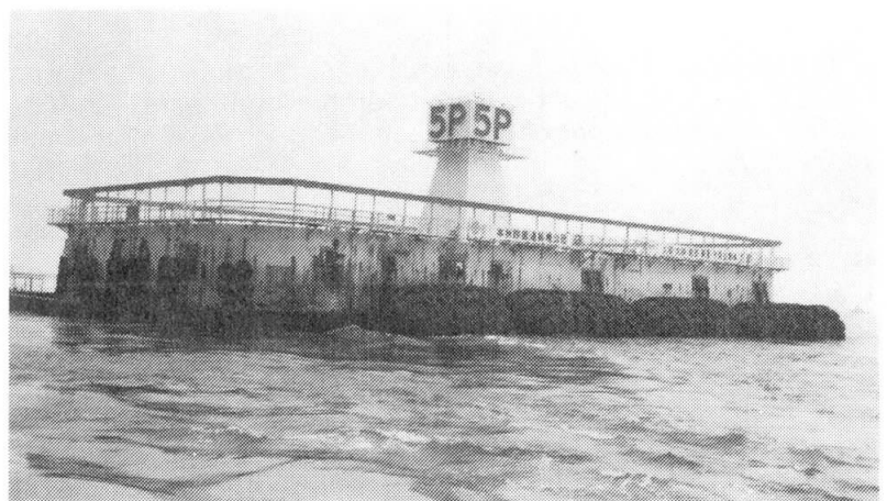
Fig.2 The Protection Installed on the No.5 Pier of the South Bisan-seto Bridge
