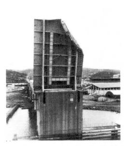
Fig 4. Damage on the Jordfallet bascule-bridge
