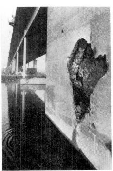
Fig 5. Damage on a bascule-pier at the Jordfallet-bridge
