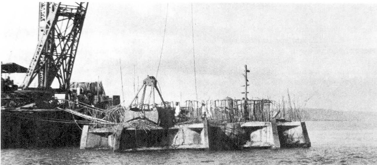
Photograph 5: Showing fender under construction.
