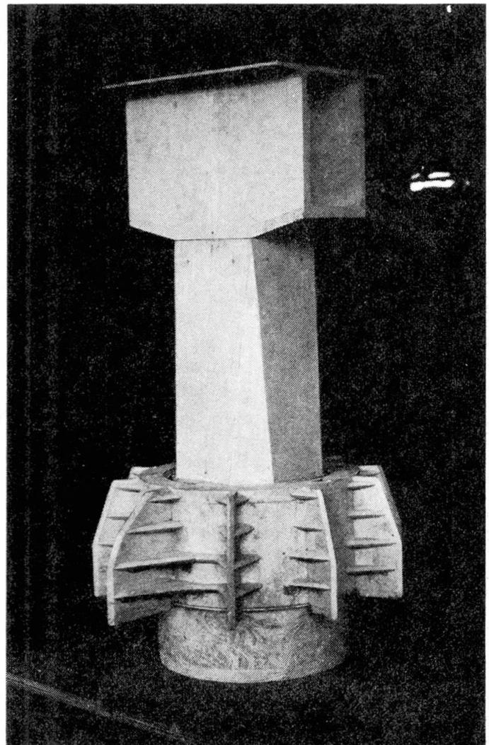
Photograph 4: Model showing section of the bridge deck, pier, fender and caisson.
