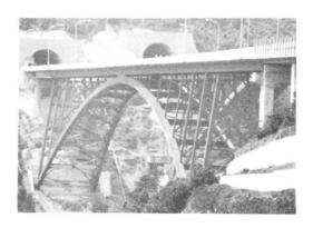
Fig.2 An arch bridge that caused lateral vibration.
