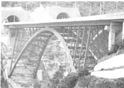
Fig.2 An arch bridge that caused lateral vibration.
