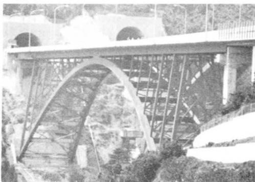
Fig.2 An arch bridge that caused lateral vibration.
