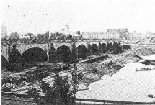
Photograph 5 : General view of cofferdam construction works.
