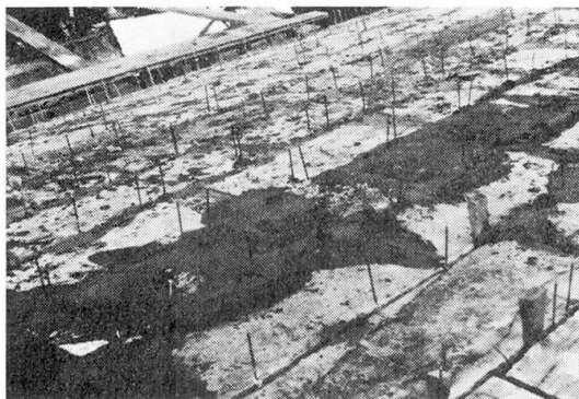
Photographs 9 & 10 : Installation of facing stones on the centre.
