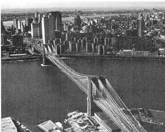
Fig.1. The Brooklyn Bridge, one of the most famous bridges in the world, celebrates its Centennial in 1983. Though no one would dream of replacing it, a cable corroded by pigeon dung snapped last year, killing a pedestrian; rehabilitation costs are estimated at \$105 million. Jack Boucher, HAER.
