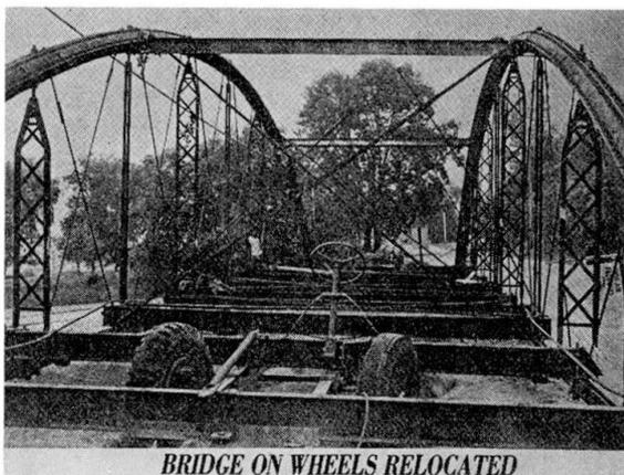
Fig.3. Espyville Road Bridge (1873), a bowstring arch-truss fabricated by the Wrought Iron Bridge Company of Canton, Ohio, was braced, lifted from its abutments, placed on a wheeled under carriage, and driven to a new location over the Olentangy River near Caledonia, Ohio - an unusual, but simple alternative to demolition.
