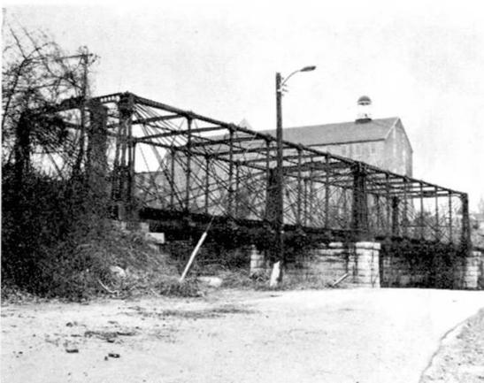
Fig.2. Bollman's Suspended & Trussed Bridge (1869) was relocated from a main line of the Baltimore & Ohio RR to service the mill at Savage, Maryland. It is the only known example of its type and facilitated the rapid expansion of early American railroads westward. Robert Vogel, Smithsonian Institution.
