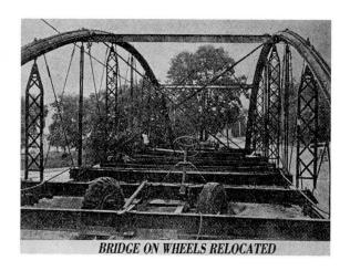
Fig. 3. Espyville Road Bridge (1873), a bowstring arch-truss fabricated by the Wroght Iron Bridge Company of Canton, Ohio, was braced, lifted from its abutments, placed on a wheeled under carriage, and driven to a new location over the Olentangy River near Caledonia, Ohio - an unusual, but simple alternative to demolition.
