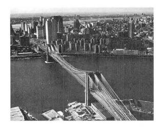
Fig.1. The Brooklyn Bridge, one of the most famous bridges in the world, celebrates its Centennial in 1983. Though no one would dream of replacing it, a cable corroded by pigeon dung snapped last year, killing a pedestrian; rehabilitation costs are estimated at \$105 million. Jack Boucher, HAER.
