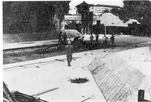
**Photograph 6 : Slab casting.**
