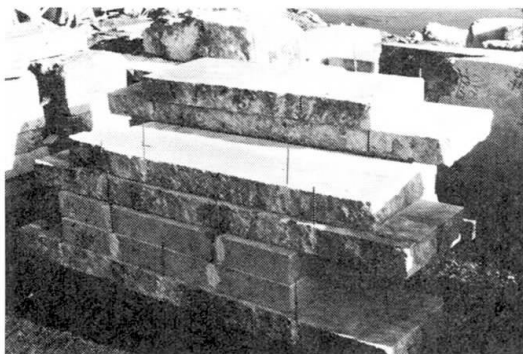
Photograph 7 : Stone facings (from the soffit)
