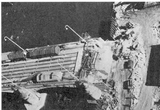
Photograph 3 : Temporary stabilization cables on the deck.
