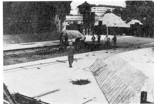
Photograph 6 : Slab casting.
