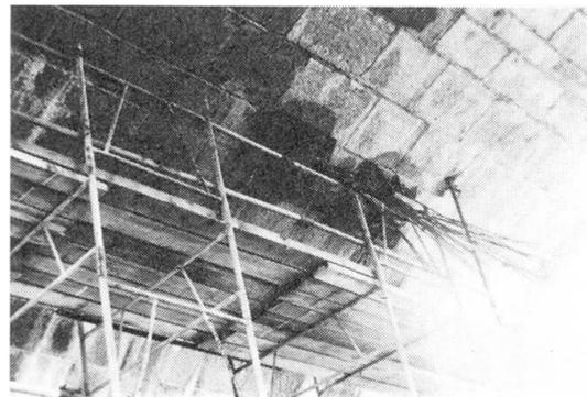
Photograph 4 : Anchorages under the 11th arch.
