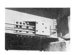
(a) POST-TENSIONING BRACKET AND TENDONS IN POSITION
