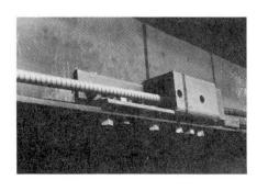
(a) POST-TENSIONING BRACKET AND TENDON IN POSITION
