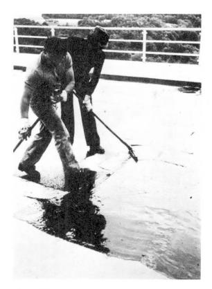
Fig. 21 Spreading of the bitumen epoxy resin waterproofing by hand (bridge over the Kocher valley at Geislingen)
