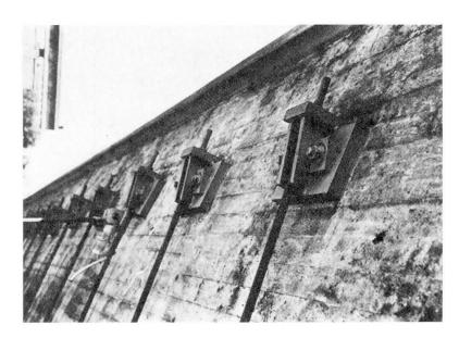
Fig. 16 Underside view with anchoring of outside additional tendons (1st rehabilitation) (Schmargendorf bridge)
