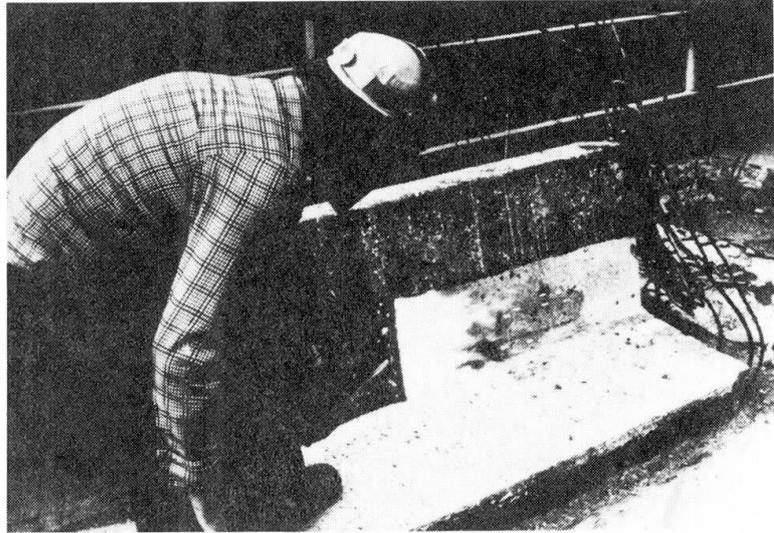
Fig. 22 Flame-cleaning of carbonated top concrete layer of concrete guard kerbs (valley bridge Pfädchensgraben)
