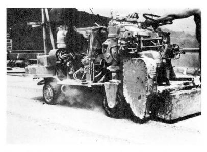
Fig. 20 Mechanical removal of carbonated top concrete layer from carriageway (bridge over the river Nahe at Dietersheim)
