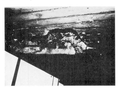
Fig. 14 Underside view of hollow box in the region of coupling joint - laid open (flyover Prinzenallee)
