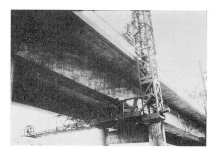
Fig. 11 Bridge inspection equipment Passarella
