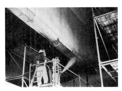
Fig. 23 Restoration of the required dimension by means of shotcrete (bridge over the river Lahn at the Taubenstein)
