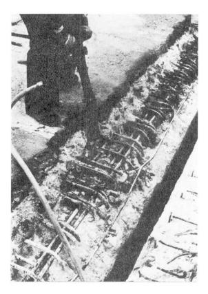
Fig. 17 Expansion joint removed (valley bridge Pfädchensgraben)
