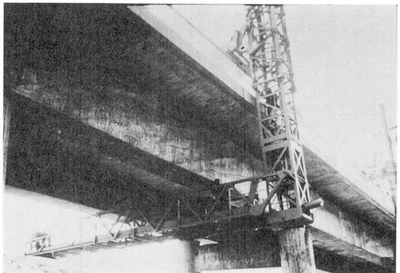
Fig. 11 Bridge inspection equipment Passarella
