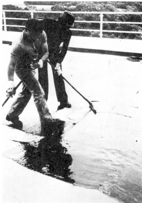
Fig. 21 Spreading of the bitumen epoxy resin waterproofing by hand (bridge over the Kocher valley at Geislingen)
