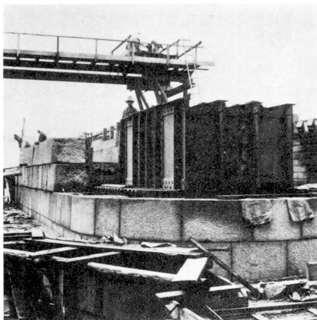
Under each pylon bearing a heavy grid of bolted steel girders of 1,60 m high was concreted into the head of the pier. For better distribution of the load the grid rested upon rolled I-beams layed closely to each other (Fig.1 to 3). No other reinforcement of the piers was provided. The external dimensions of the pier shaft were just so large that the steel grid and the mat of rolled beams found enough
