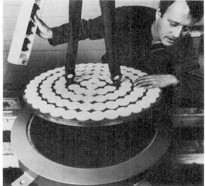
**Fig. 9** Assembly of a Sliding Pot Bearing
