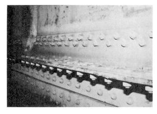
Figure 11 Repair to bottom of web
