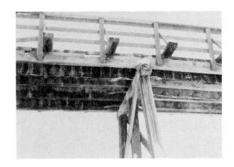
Figure 2 Crushing Timber
