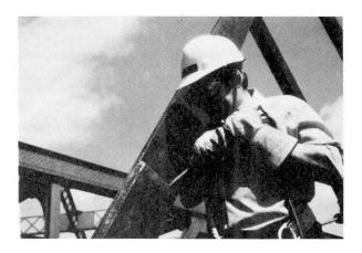
Figure 19 Peening welds
