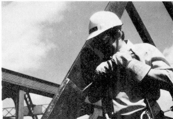
Figure 19 Peening welds
