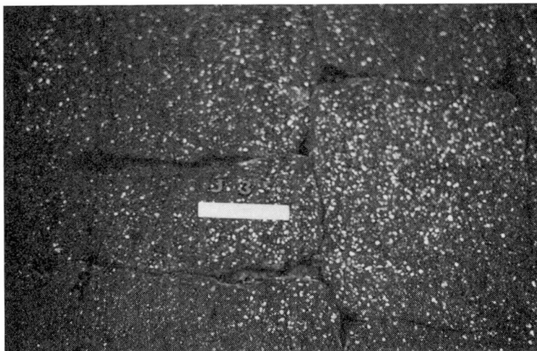
Fig. 3 Severe Cracking of the Surfacing
