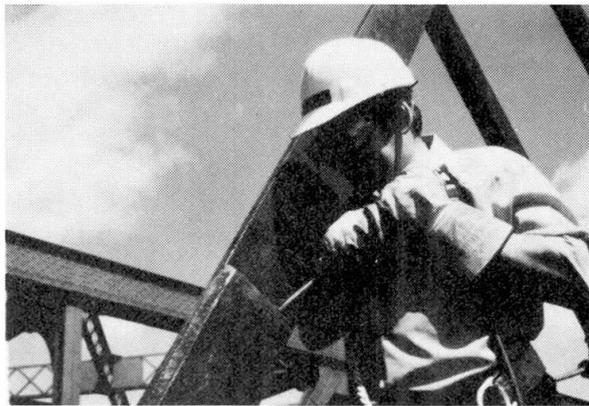
Figure 19 Peening welds
