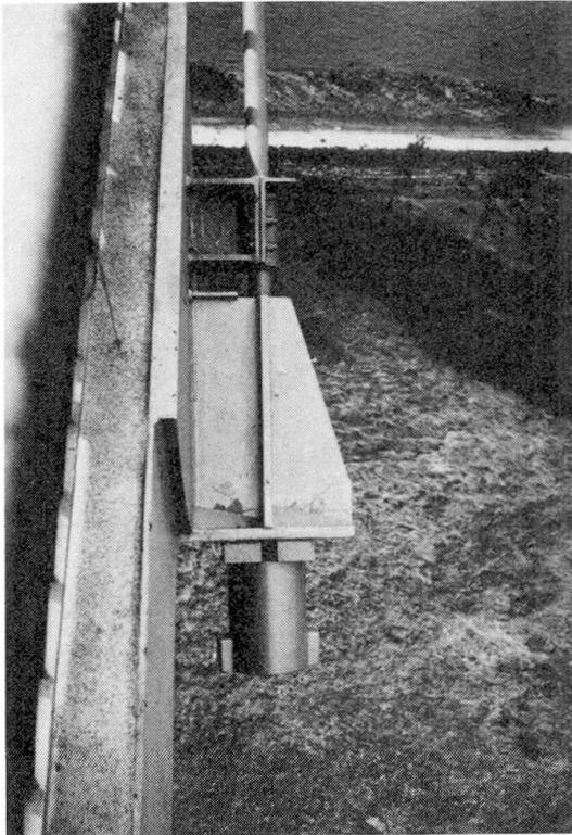
It stands to reason that damping devices should be installed wherever dynamic effects can be presumed to have adverse effects on the life expectancy of cables or where the behaviour of an existing bridge suggests that damping devices are installed as a rehabilitation measure. Fig. 8 and 9 present examples of possible solutions for the installation of damping devices as a rehabilitation measure. The spring-type dampers as shown on Fig. 9 were fixed to stiffened hand rails.
