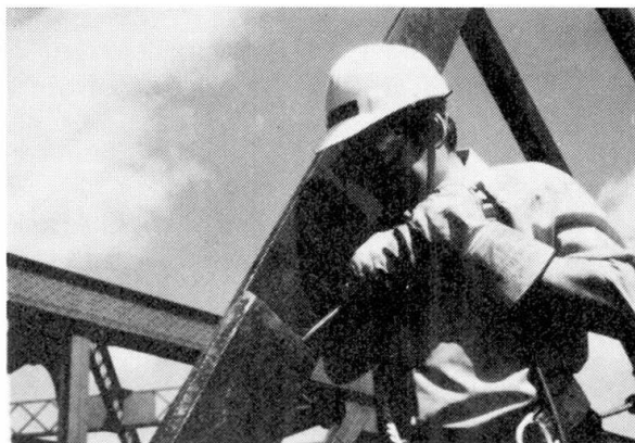
Figure 19 Peening welds
