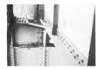
Figure 18 Bracing leads nowhere
