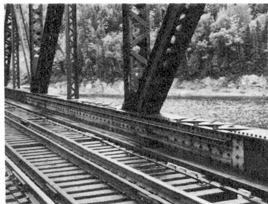
Figure 12 Member spliced
