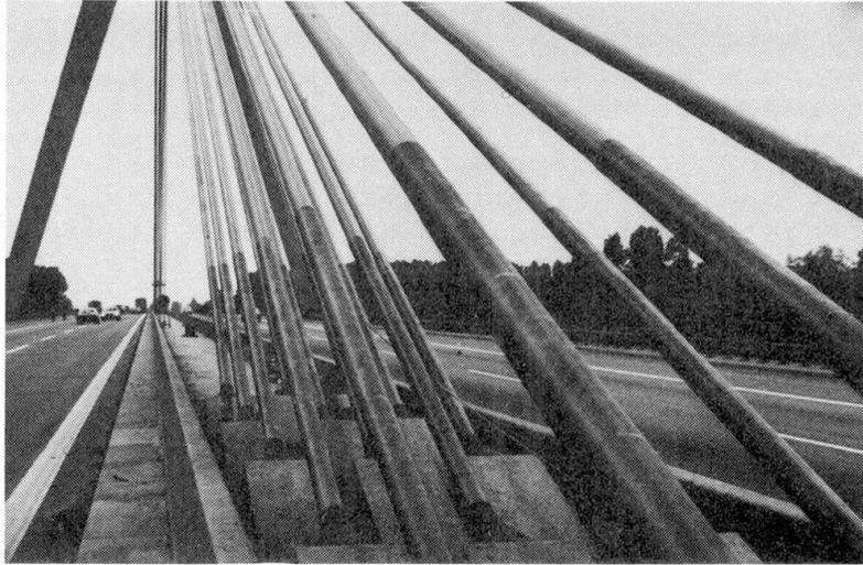
Fig. 11 Additional Wrapping in Splash-Zone
