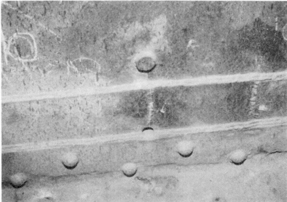
Figure 3 Crack in Girder
