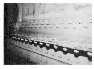
Figure 11 Repair to bottom of web
