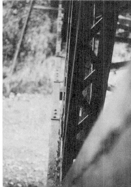
Figure 13 Broken welds
