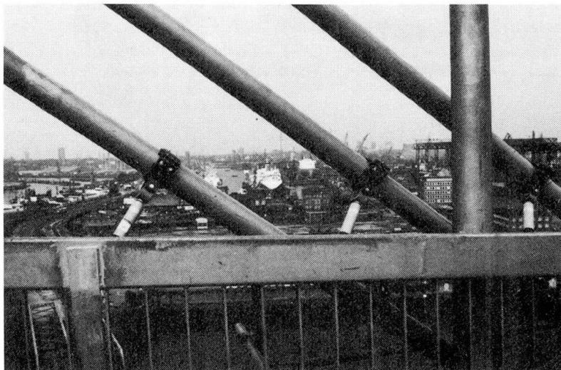
Fig. 9 Spring Type Damper
