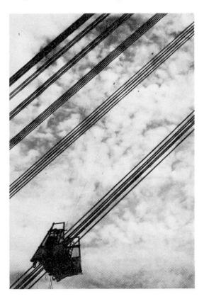
Fig. 10 Inspection of Cables
