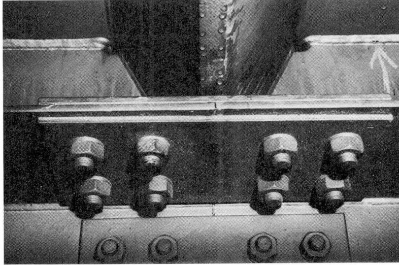
Fig. 2 Dew-Drops on the Underside of Stiffeners
