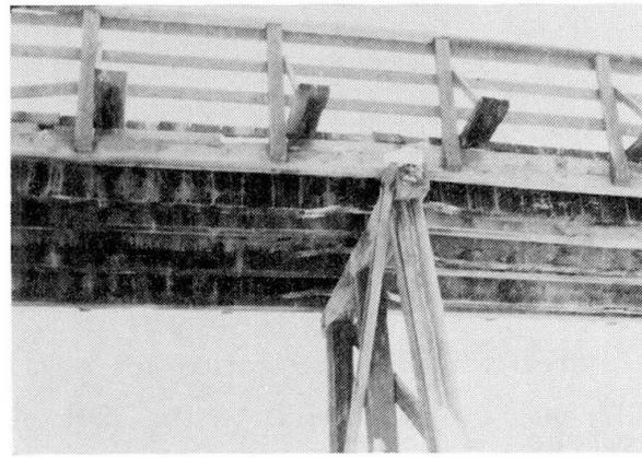
Figure 2 Crushing Timber
