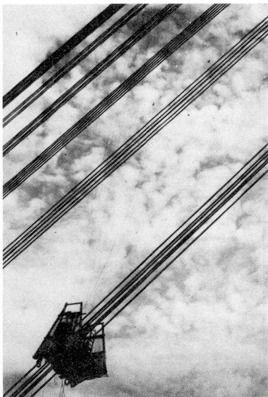
Fig. 10 Inspection of Cables
