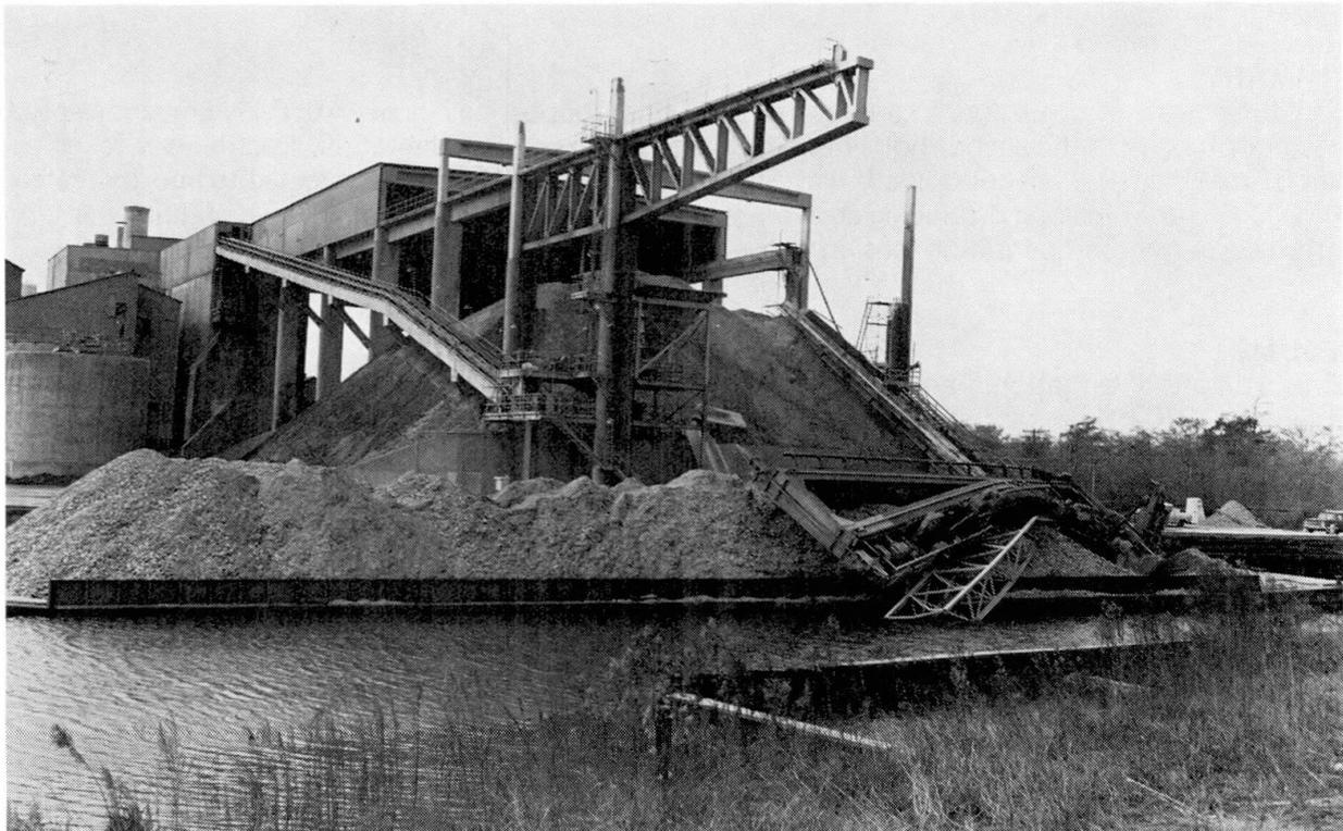
Fig. 1 View of Collapsed Truss and Crane
