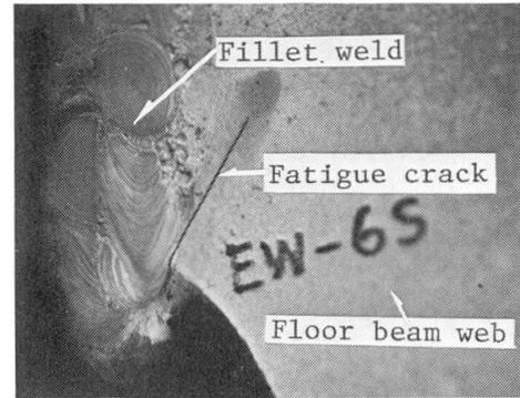
Fig. 6 Fatigue crack in floor beam web
