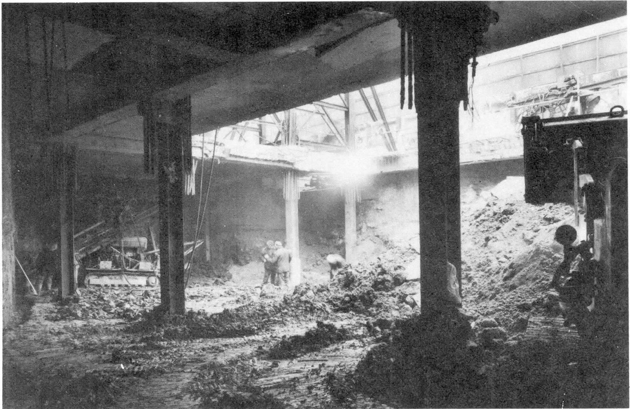
Fig 1 Ground anchor installation and excavation beneath the ground floor slab of a basement substructure, Victoria Street, London
