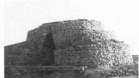
Fig 2 Corbelled arch
