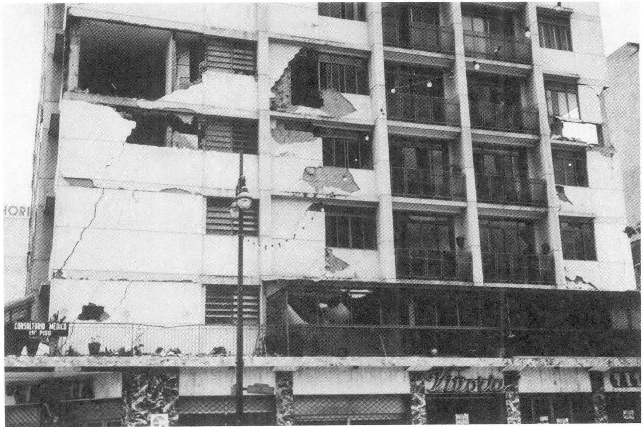
Fig. 10: Damage to nonstructural elements in 1967 Caracas, Venezuela earthquake
