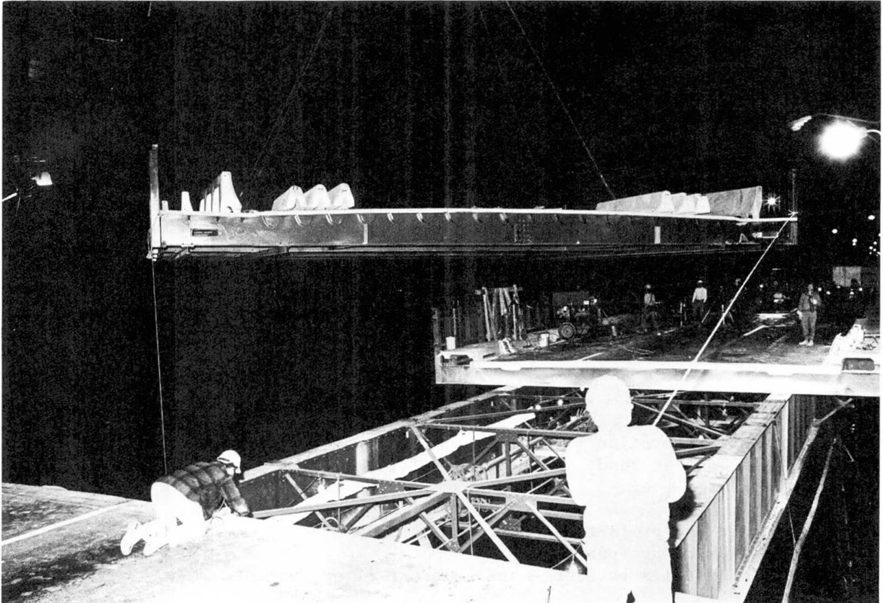
Fig. 8 Section of North Viaduct during Installation.
