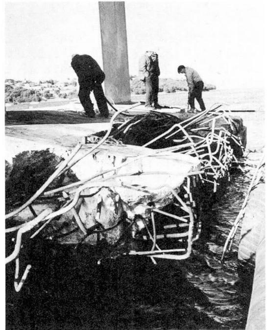
Fig. 5 Damage to Pile Cap 20
