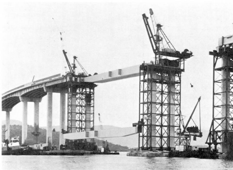
Fig. 11 Box girder erection
