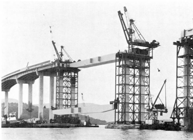
Fig. 11 Box girder erection
