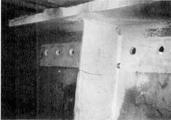
Fig. 11 Hole at Stiffener
