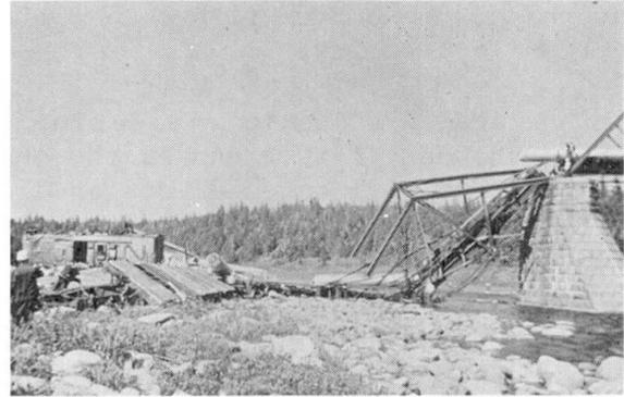
Fig. 15 Insufficient Redundancy
