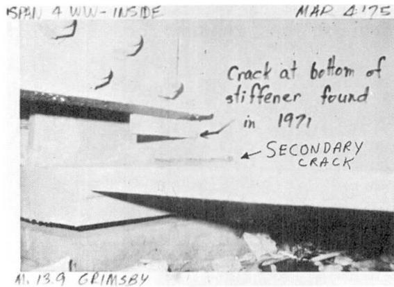
Fig. 5 Secondary Cracking
