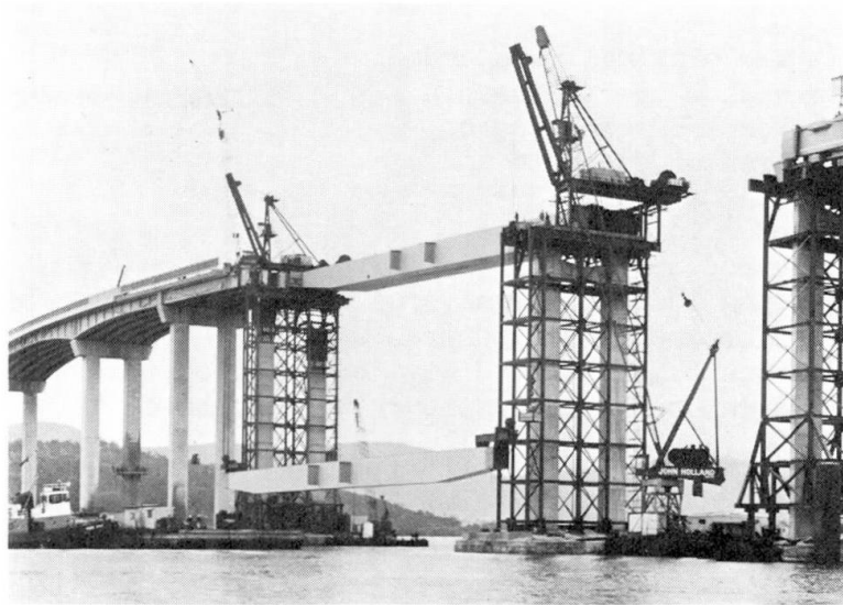
Fig. 11 Box girder erection
