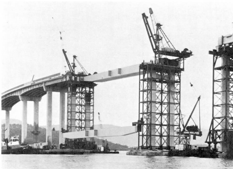
Fig. 11 Box girder erection
