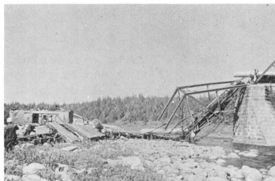
Fig. 15 Insufficient Redundancy
