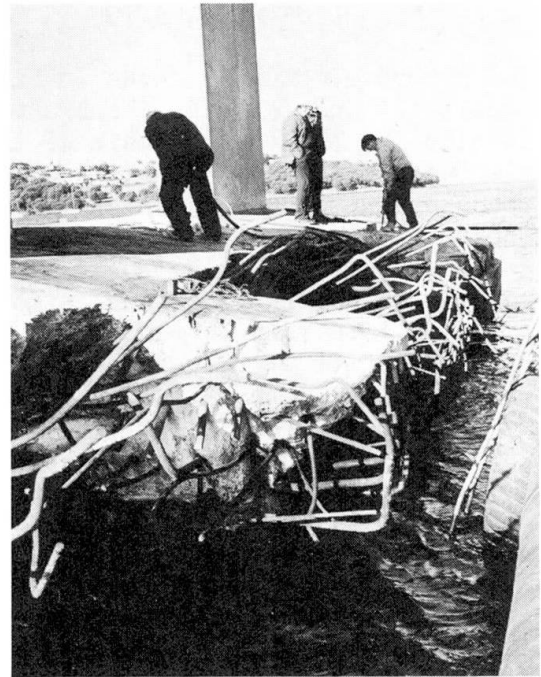
Fig. 5 Damage to Pile Cap 20
