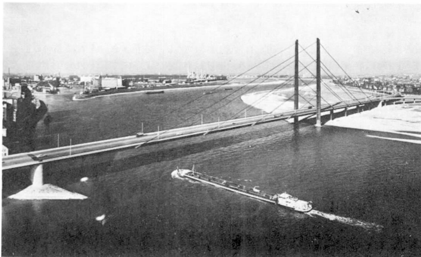
Fig. 4 Long-Span Bridge; Kniebrücke-Rhine River, W. Germany
