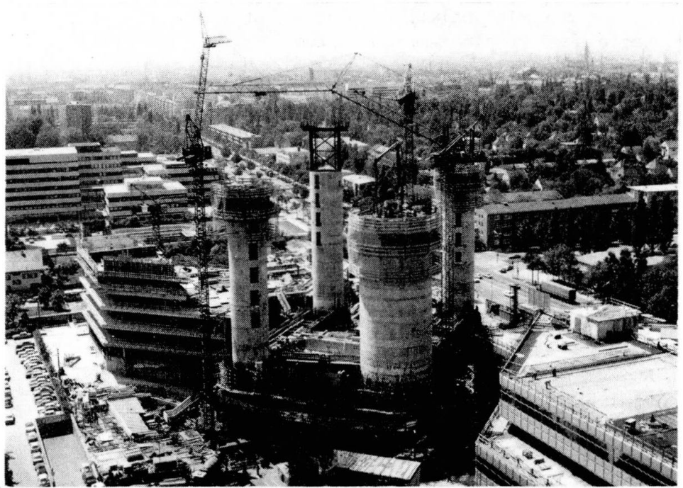
Fig. 1 View of building site
