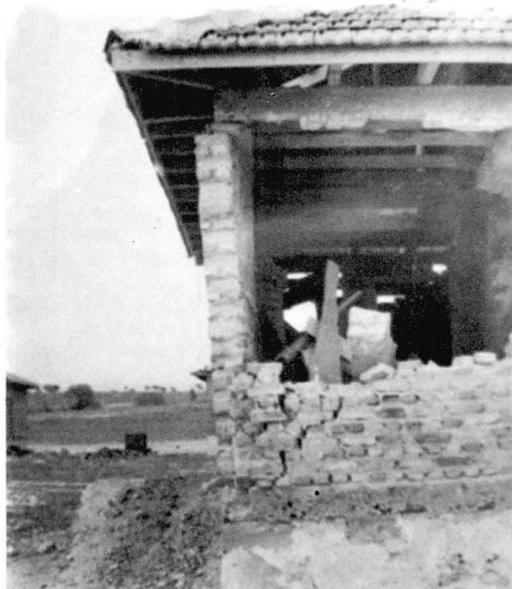
Figure-3 Corner Damage due to Earthquake
