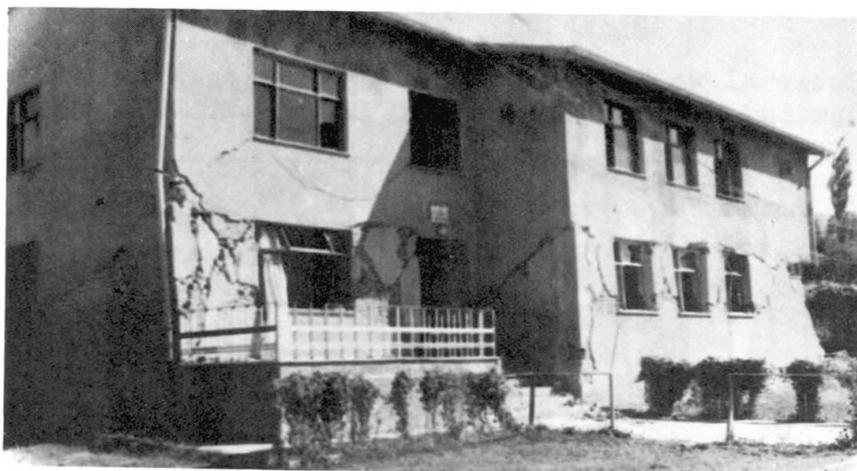
Figure-6 Typical Failure of Brick Masonry
