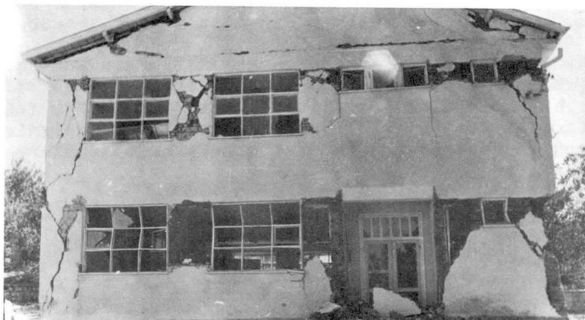
Figure-5 Typical Failure of Brick Masonry
