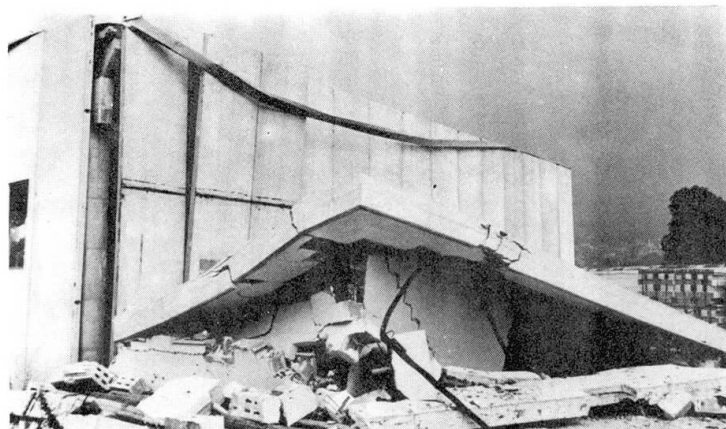
Figure 4: (after September 15th): Prefabricated shed with collapsed annex. The renewed earthquake load caused damage of the supporting framework of the shed at the fixing points of the columns and rests of the bars. The façade slabs of the side wall were severely caved in by the renewed impact: the annex itself collapsed. The increased displacement, as compared with the first earthquake, can be traced back to the reduced structural rigidity due to the destruction of one of the concrete block walls.
