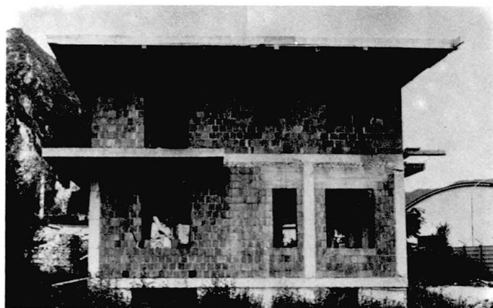
Figure 1: (after May 6th): Uncompleted building in Gemona with groundfloor open on three sides and living floor above. The supporting framework of the groundfloor consists of reinforced concrete columns, partitioned on one of the narrow sides by brick walls. The upper floor is exclusively brick. Due to the earthquake load, the building rotated around the partitioned transverse wall in the groundfloor. The fixing points of the columns were badly damaged in the cellar and groundfloor ceilings. The brick walls on the transverse side on the groundfloor were slightly cracked: the upper floor remained undamaged.
