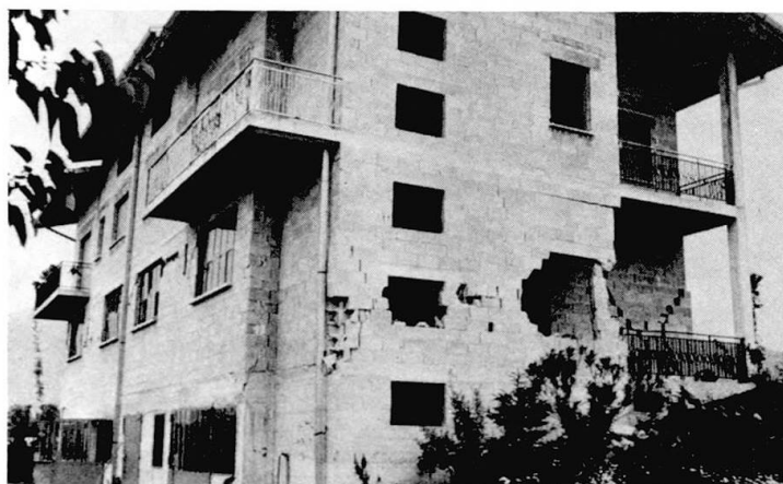
Figure 5: (after May 6th): Residential building with workshop near Artegna with a reinforced concrete cellar and two floors in concrete blocks. The side walls by the entrance incurred gaping X-shaped diagonal cracks due to the high shear stress. These cracks led to partial collapse of the masonry. The highly strained window jambs on the longitudinal façade were badly cracked.
