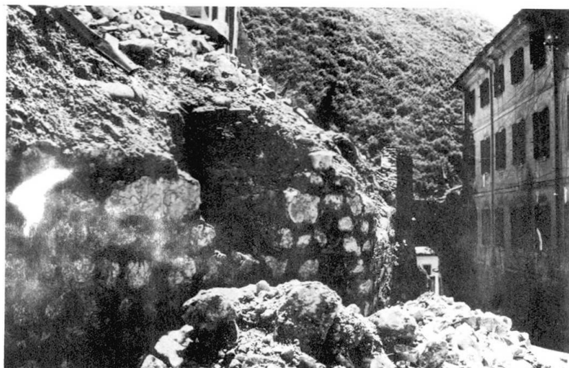
Fig. 7. Duomo Gemona; Failure of the retaining wall.
