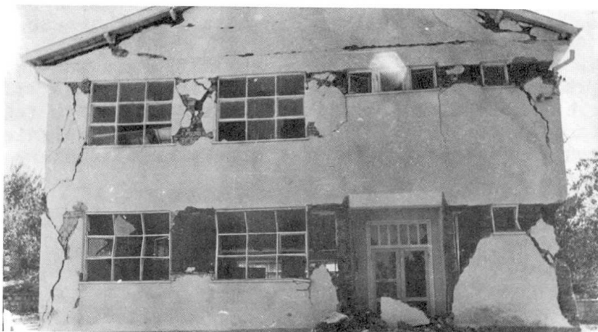
Figure-5 Typical Failure of Brick Masonry
