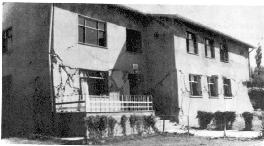
Figure-6 Typical Failure of Brick Masonry
