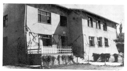
Figure-6 Typical Failure of Brick Masonry
