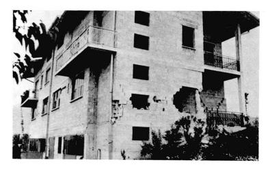
Figure 5: (after May 6th): Residential building with workshop near Artegna with a reinforced concrete cellar and two floors in concrete blocks. The side walls by the entrance incurred gaping X-shaped diagonal cracks due to the high shear stress. These cracks led to partial collapse of the masonry. The highly strained window jambs on the longitudinal façade were badly cracked.
