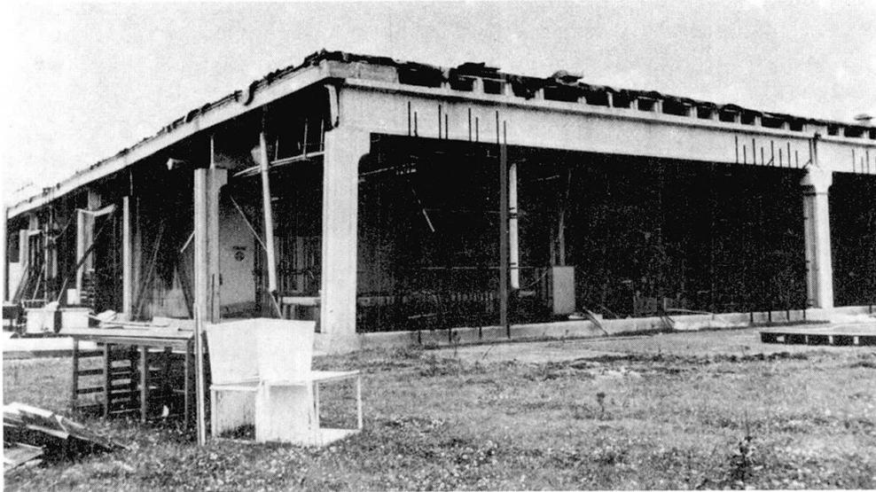
Figure 11: (after May 6th): Factory building near Artegna. Severe displacement of the prefabricated reinforced concrete framework together with distortion of the foundation and tilting of a corner column. A large number of the only lightly secured reinforced concrete façade elements were thrown off.
