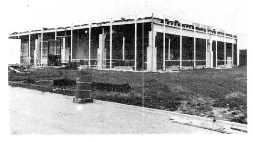
Figure 12: (after September 15th): Factory building near Artegna, after repair, without further earthquake damage. In order to increase the carrying capacity, the concrete columns were surrounded with a 15 cm strong concrete sheath. The earthquake load was reduced by replacing the heavy concrete façade elements by a Tight metal façade.
