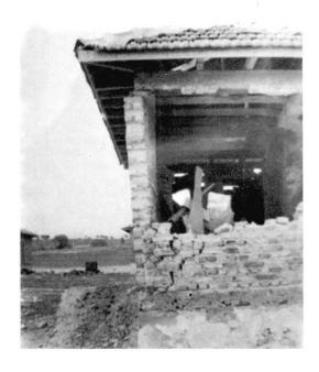
Figure-3 Corner Damage due to Earthquake
