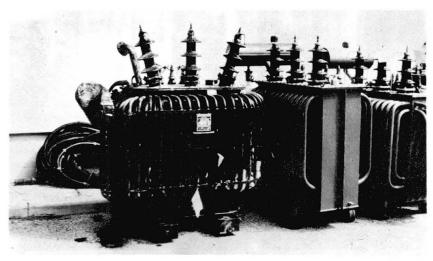
Fig 1. Damaged and new distribution transformers.
