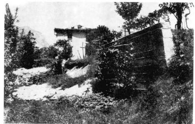
Fig. 7. Duomo Gemona; Failure of the retaining wall.
