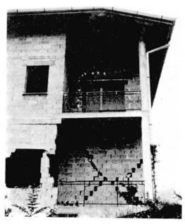
Figure 13: Dwelling house with workshop near Artegna. Basement in reinforced concrete and the upper stories in masoning without framing. Typical diagonal cross cracks in a wall of the ground floor.
