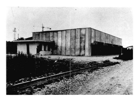
Figure 16: Prefabricated storage shed with brick annex in Gemona. Side wall panels slightly caved in by impact with rigid annex. Upper part of the annex shorn off and pushed over by the impact force due to insufficiently wide joints.
