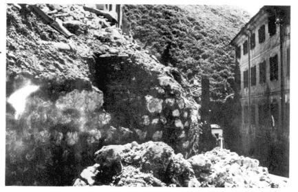
large as in the valley. The slip vectors, however, were large enough to cause the failure of retaining walls. Figure 6 was taken from Gemona. The low strength masonry wall could not resist the slip vector as did the concrete wall sitting next to it.
