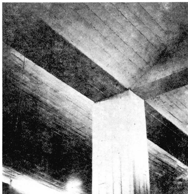
Fig. 7 - Detail of main frame joint
