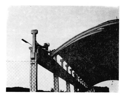
Fig. 10 (above) Industrial hangar at Magnano; collapse mechanism.
