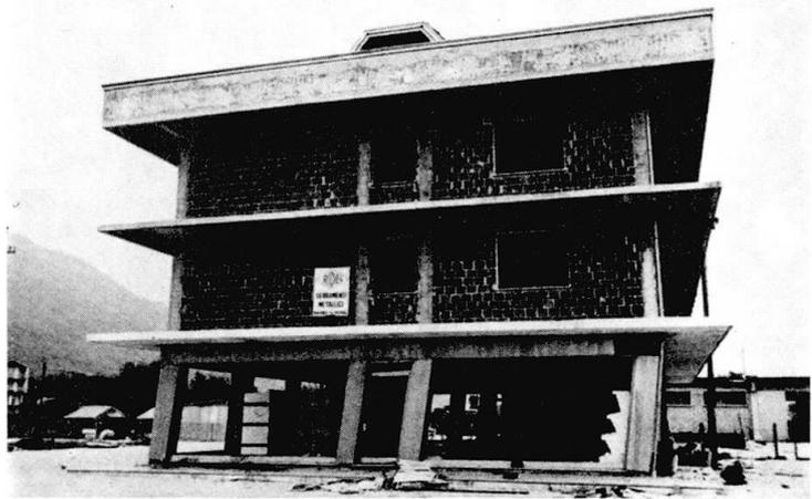
The ground plan of the dwelling house with the open ground floor shown before. Twisting of the building around the staircase stiffened with masonry walls.
