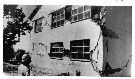
Figure-7 Typical Failure of Brick Masonry
