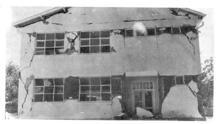
Figure-5 Typical Failure of Brick Masonry
