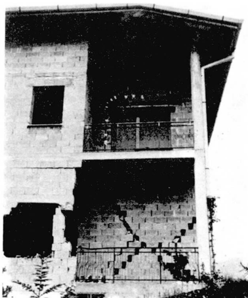
Figure 13: Dwelling house with workshop near Artegna. Basement in reinforced concrete and the upper stories in masonry without framing. Typical diagonal cross cracks in a wall of the ground floor.
