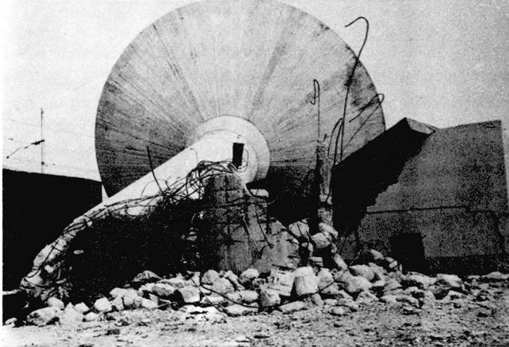
Figure 17: Overturned water tower belonging to the Italian State Railways in Gemona station. Foot of the shaft completely destroyed and concrete shattered.
