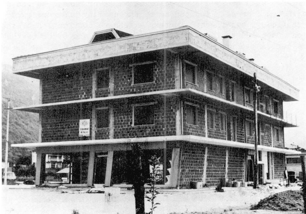
Figure 7: (after May 6th): Residential building with shop near Artegna. Reinforced concrete frame building with brick partitioning in the two upper storeys. In the groundfloor, open on three sides, only the rear longitudinal wall and the staircase are braced. The destruction was concentrated on the groundfloor where a rotating motion of approximately 40 cm maximum displacement occurred around the staircase core. The brick walls of the staircase were badly destroyed, while those of the upper floors remained undamaged.
