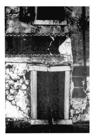
Fig. 8 Collapse mechanism of masonry wall at Gemona.
