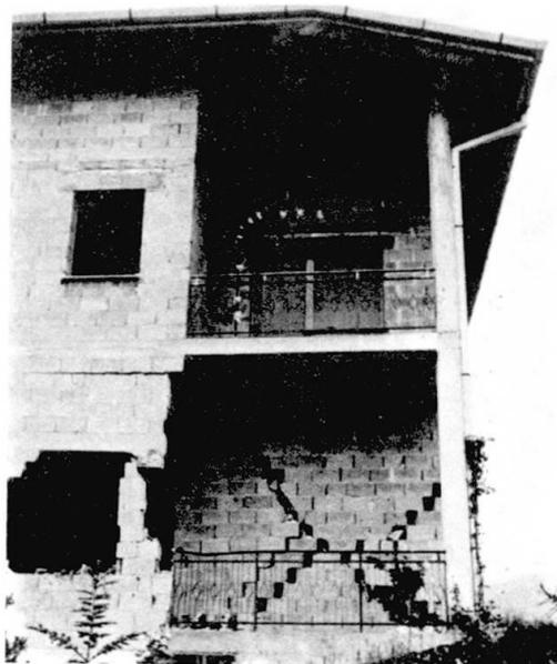
Figure 13: Dwelling house with workshop near Artegna. Basement in reinforced concrete and the upper stories in masonry without framing. Typical diagonal cross cracks in a wall of the ground floor.
