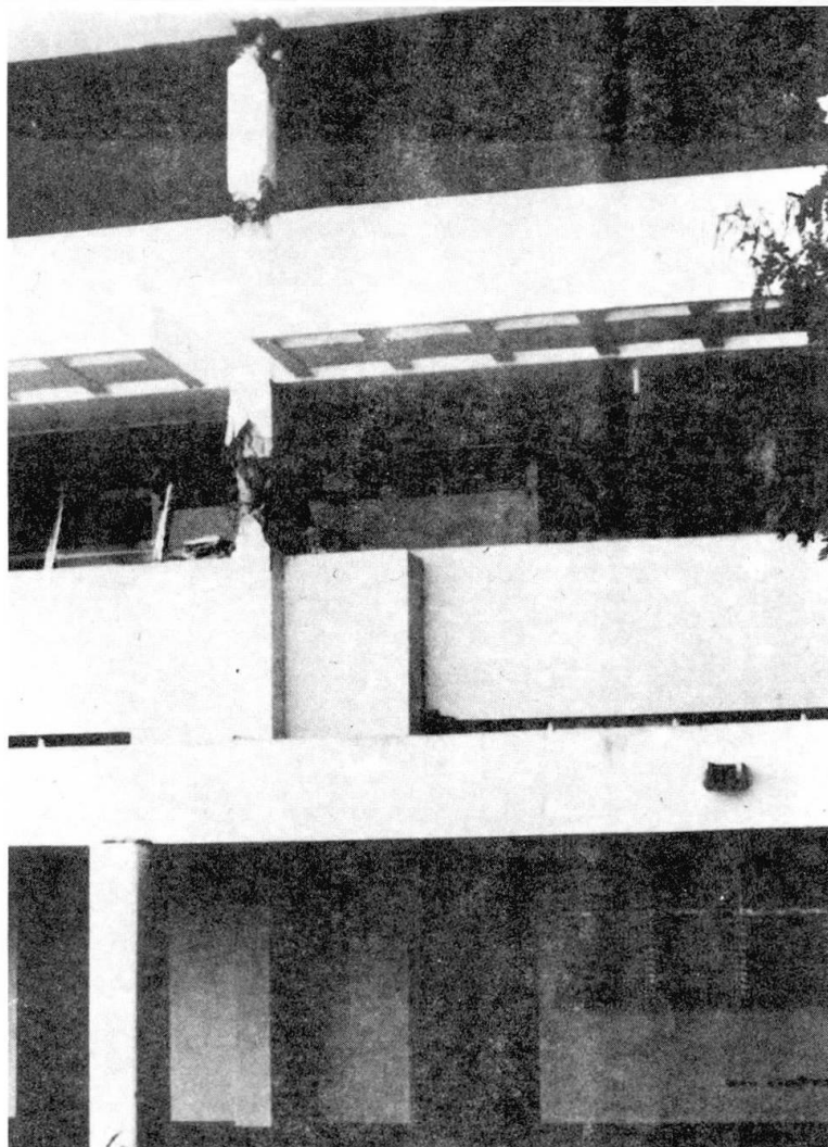
Figure 1. Colegio Teresiano in Managua, Nicaragua, after 1972 earthquake. First story stiffening wall, which can be seen projecting outward from second floor beam, prevented first story damage but increased upper story damage.
