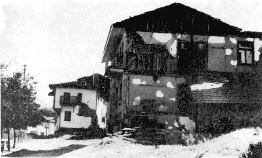
Figure 4. Typical Wood Frame Structure (Hımsı)
