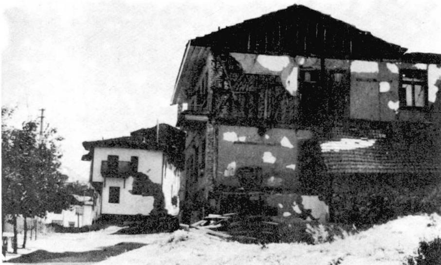
Figure 4. Typical Wood Frame Structure (Hımsı)
