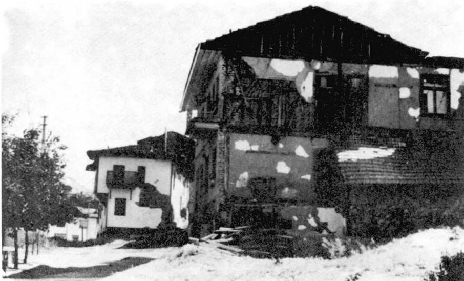
Figure 4. Typical Wood Frame Structure (Hımsı)
