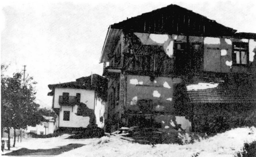
Figure 4. Typical Wood Frame Structure (Hımsı)
