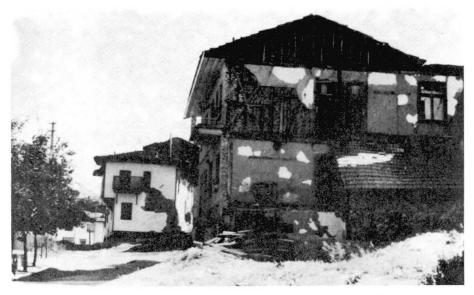
Figure 4. Typical Wood Frame Structure (Himis)
