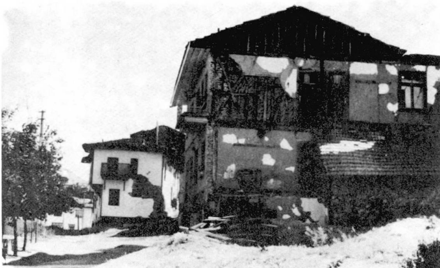
Figure 4. Typical Wood Frame Structure (Hımsı)
