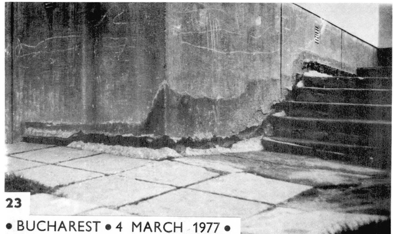
COLUMN UPLIFT DURING SEISMIC RESPONSE OF BUILDINGS
