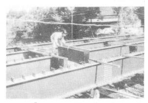
Fig. 11 Erection of U-shape Steel Form
