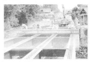
Fig. 12 Setting of I.B GRATE Floor
