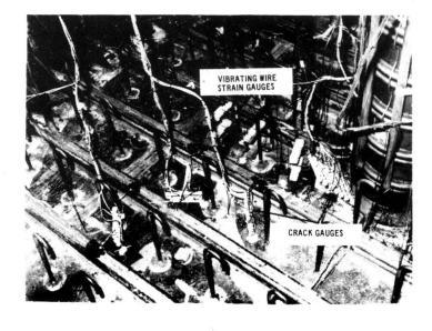
FIG. 4 VIEW OF MODEL DURING CONSTRUCTION, SHOWING INSTRUMENTATION
