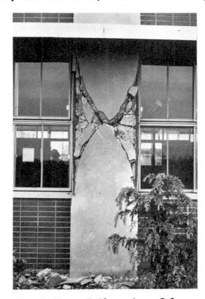
Fig. 2 Shear Failure in a Column
