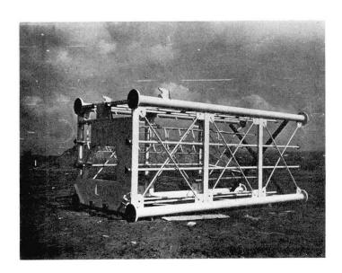
Fig. 2. Standard Section of a television mast.
