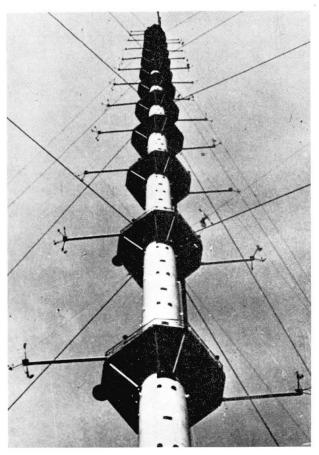
Fig. 3. Mast shaft made of steel plates.
