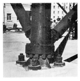
Fig. 4. Standard support tower chord-to-foundation connection.
