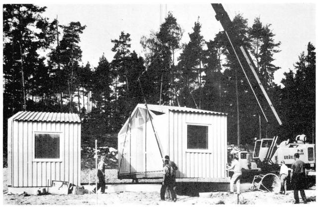
The house sections are delivered quite complete from the factory. Inner walls, partitions and wall papers, ceilings, inner floors and floor covers, cupboards and kitchen equipments, dishing and washing machines, heating, ventilation, sanitary and electrical equipment are all installed on the assembly line in the factory. All sections are structurally the same and made in the same way but furnished with different equipment.
