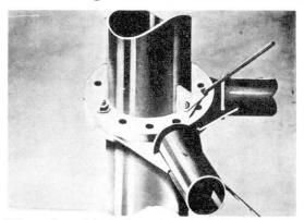
Fig.1. Standard field joint in the tower chords with prestressed diagonals.
