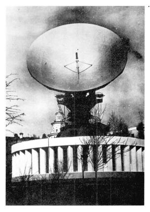
Fig. 5. Standard full revolving antenna 12.0m dia.
