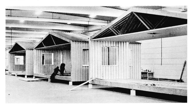
All sheet steel is galvanized to 30  $\mu$ m zink thickness and all outer surfaces are plastic coated with 200  $\mu$ m Organosol. The plate thickness is 0,9 mm and the height of the trapezium-profile pattern is 45 mm.
