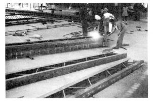
$$\operatorname{Fig}\ 15$$  Assembly of a complete portal
