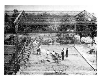
$$\operatorname{Fig}\ 6$$  Prototype testing of portal frame
