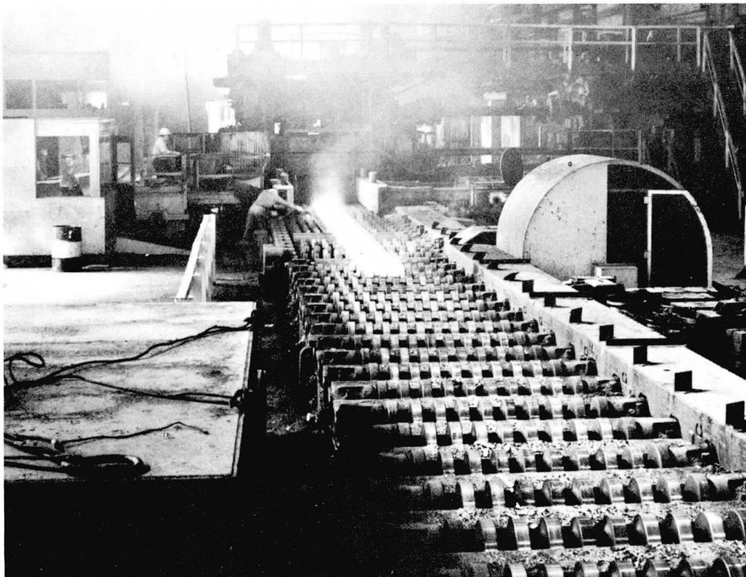
Fig. 5 The Rolling of Thick, Heavy Plates.
