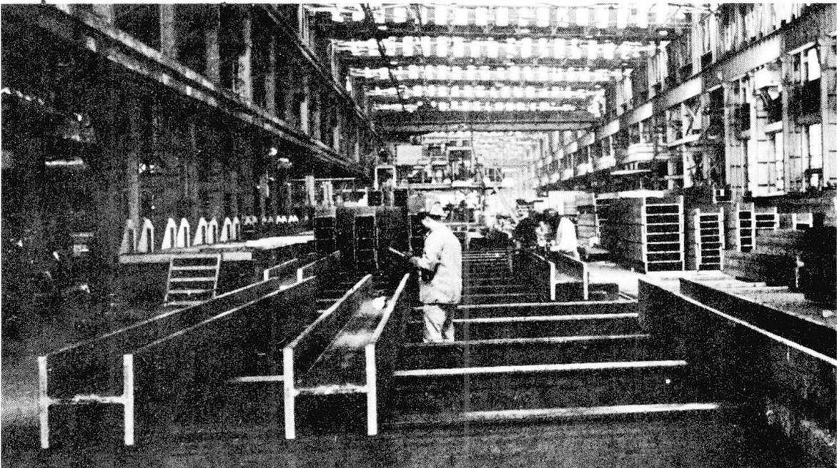
Fig. 11 Inspection Skids (Courtesy Inland Steel Company)
